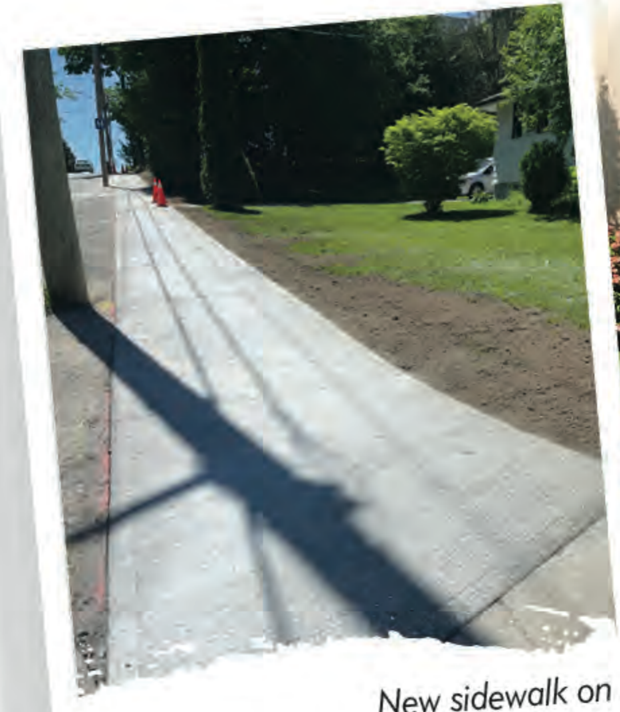
New sidewalk on Dublin Street, Mount Forest.
