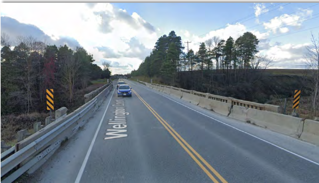
Looking west over C109123
