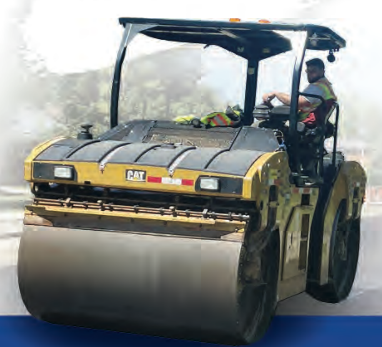
Paving of the newly reconstructed Smith Street in Arthur.
